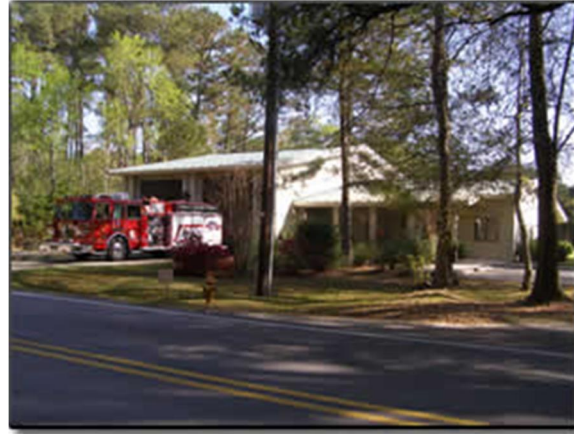
Fire Station #32 - Callawassie
