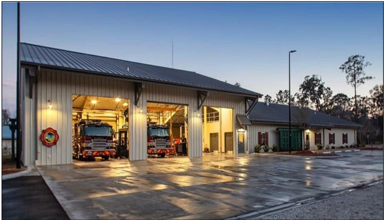
Bluffton Township Fire District Maintenance and Training building.
