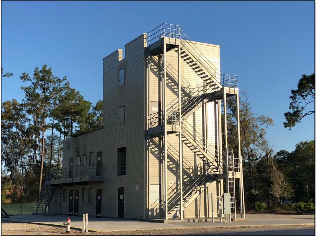
Bluffton Township Fire District Training Tower and burn building.
