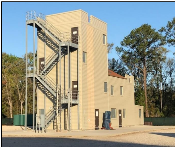
Bluffton Township Fire District Training Tower and burn building.
